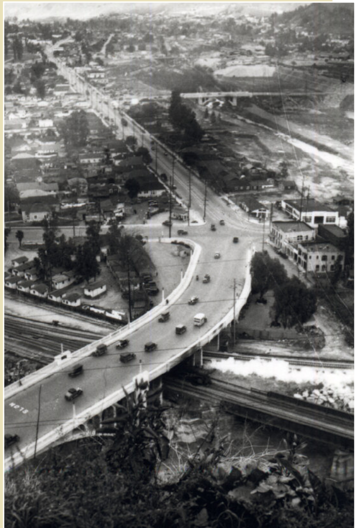
Highway over rail yards, Los Angeles, 1934.
